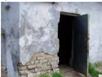
Entrance to the Gagarinsk orphanage's facilities before renovation...
